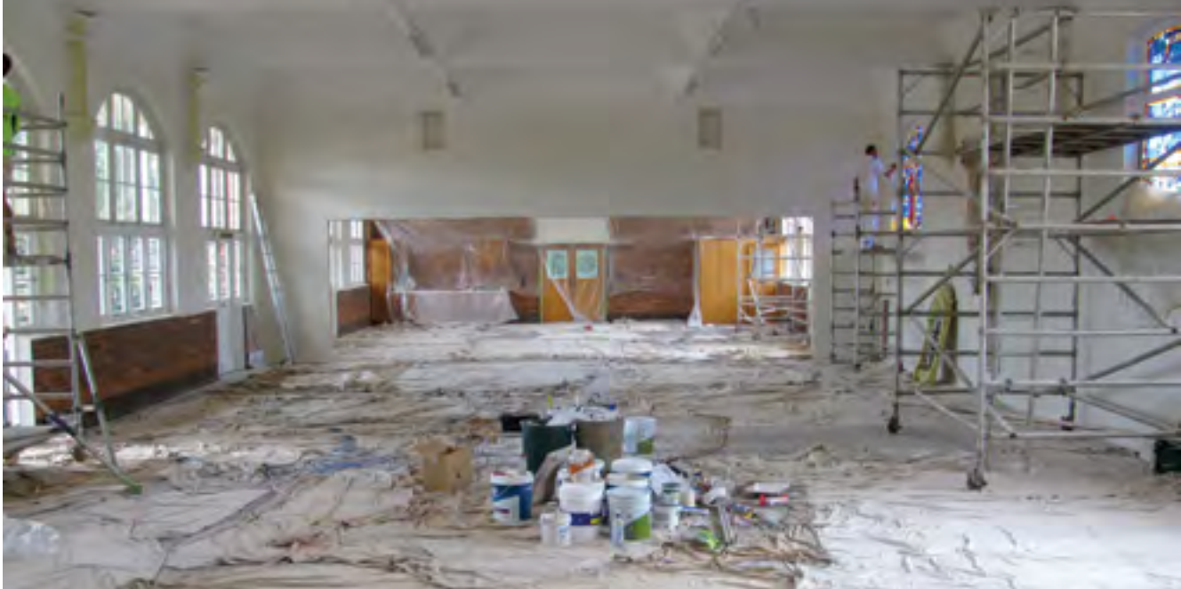
The Church empty and ready for painting.
